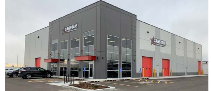
Previous examples of TAG Developments build-to-suits
